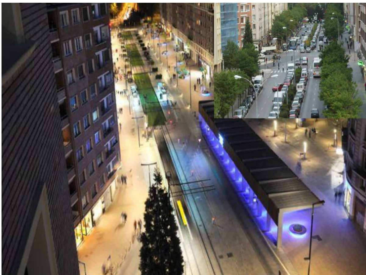
Implemented superbloc in Vitoria-Gasteiz; Sancho el Sabio Street. Before and after.
